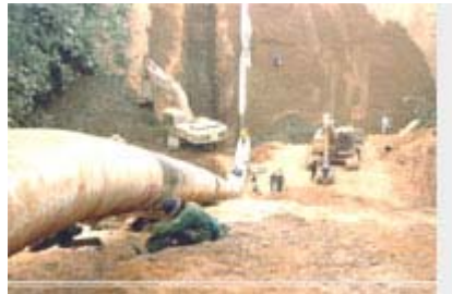
Laying the pipeline on uneven terrain
