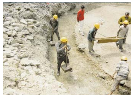
Laying of concrete base for a clear water reservoir in Nainital
