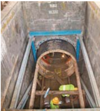
Construction of a 200 meter long DIA segmental tunnel boring at Jessore Road
