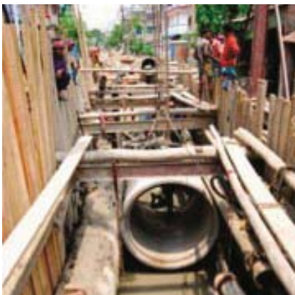
Laying of a 1600 m DIA pipe near Bama Charan at Raja Ram Mohan Roy road
