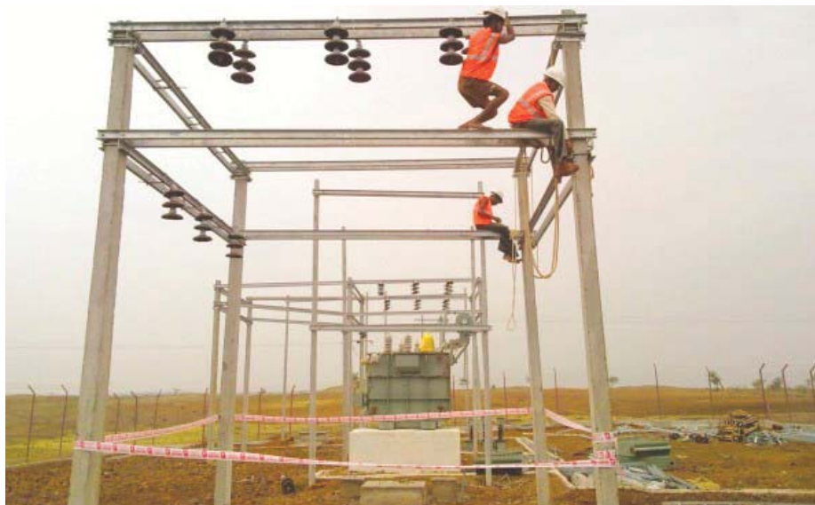
New 315 MVA 33/11 kV sub-station (and a 33 kV bay) under construction at village Kalibawdi under Dhar District of M.P. Discom West under ADB Loan No. 2520
