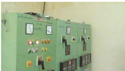
11 kV control panel in control room of a new 315 MVA 33/11 kV sub-station at Bhawarasala in Dhar district of Madhya Pradesh Discom West under ADB Loan No. 2347
