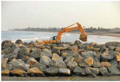
Breakwaters constructed at Nagapattinam port with disaster-resistant technology help to provide protection for vulnerable coastal communities
