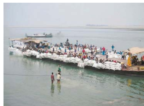
Mar 2013. Gumi Subproject area: Ongoing Cost-effective underwater riverbank erosion protections works with systematic sand-filled geo-textile bags dumping.
