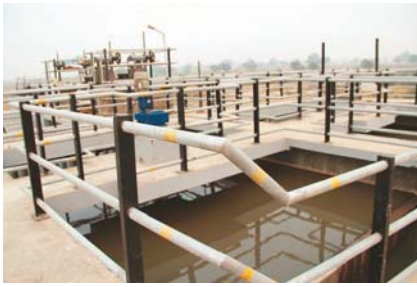
A 20 MLD waste stabilization pond type STP created in Alwar, one of the first project cities. Proper wastewater management is expected to gain momentum through creation of such assets. This is expected to reduce direct discharge of wastewater into water bodies, thereby, reducing their contamination.
