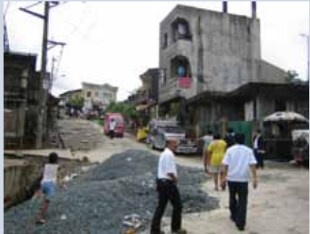
Improving road infrastructure Source: F. Steinberg.
