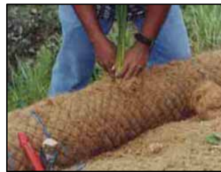
Plate 20. Section View of Coir Fiber Log Installation
