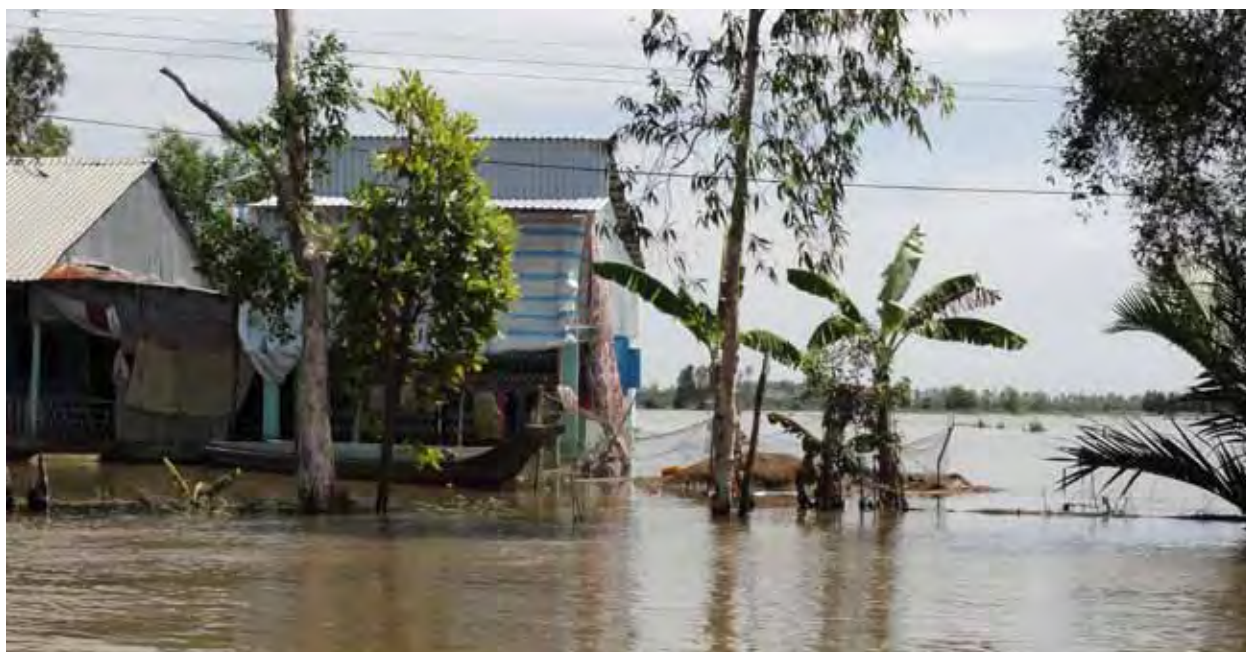
Flood waters overtopping a canal bank, inundating housing and rice fields in Hon Dat.
