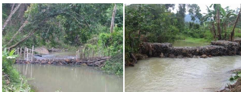
Figure 10. Wooden dam (left) and semi-permanent stone dam (right).
