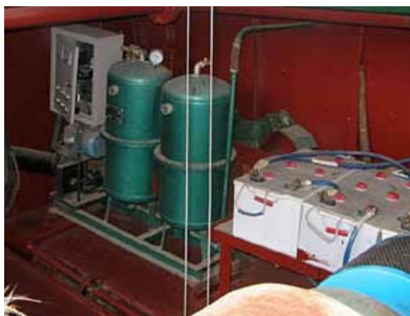
Figure 21: Oil-water separator on board cargo barge
