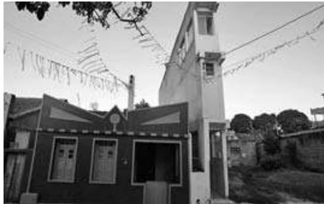
Figure 1. “Toothpick” ( palito ) house in Madre de Deus city, State of Bahia, Brazil: a six-people family lives in the ‘toothpick’ house. The building is 1.1m wide in front, 3m wide in the back, about 16 meters long and 11 meters high. “It took us three years to build the house, but this was not due to lack of a blueprint; it was for pure lack of money, actually. Practically, one year per storey”. [Source: g1.globo.com]
