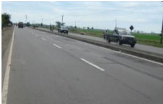
a) Notable difference in condition between lanes
