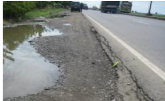
b) shoulder drop-off and poor shoulder condition
