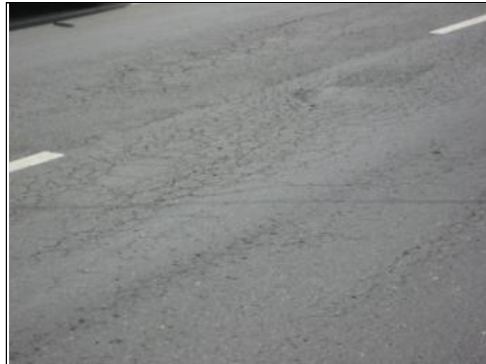
Figure 13: Photo of a Failed Section on the Trengguli PBC Area (Rutting becoming visible)
