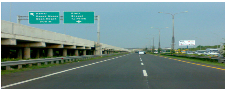
Figure 15. The toll road to the Soekarno-Hatta Air port in Jakarta has been raised up to 1.2 meter (left due to 'rhob' flood hits northern Jakarta more frequently after mangrove have been cleared (Photo: Ita Sualia, 2010)
