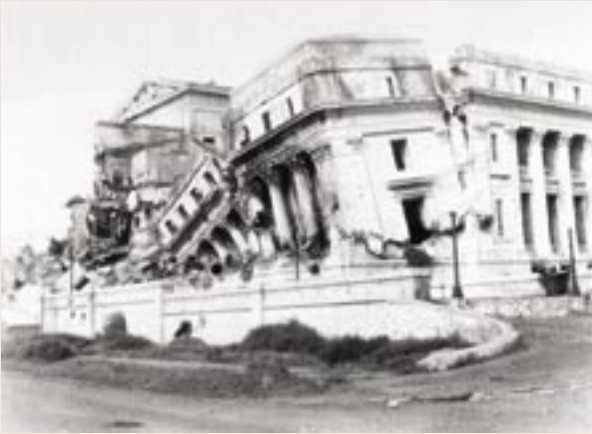
The Senate building was severely damaged by American soldiers to flush the Japanese holdouts.
