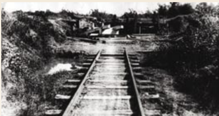
The cannon emplacement at Malinta (above) and at Malabon (below) control disrupted rail services.
