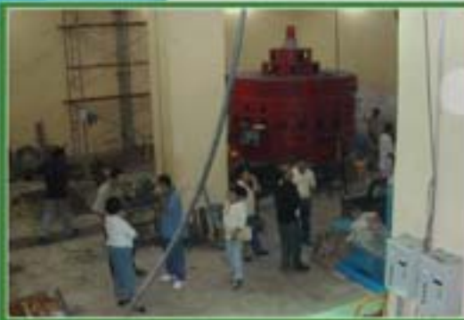
Sevilla mini-hydro power plant in Bohol, showing one of the "Two units (2 x 1250 KW) Vertical Flexible Kaplan turbines" connected to a two units (2x1250 KW) 6600 Volts, 60Hz Synchronous Generators and associated controls.
