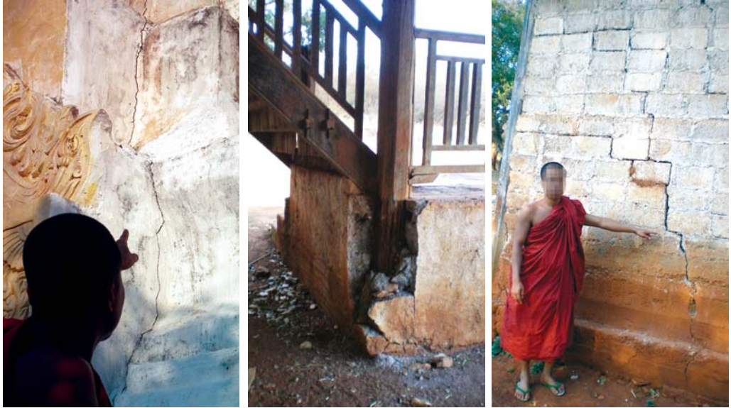
Local monks show temple walls cracked by explosions from mining for construction materials. Photos taken in March 2008
