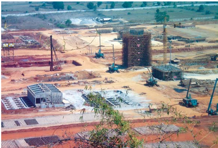
Pinpet iron factory under construction in February 2009
