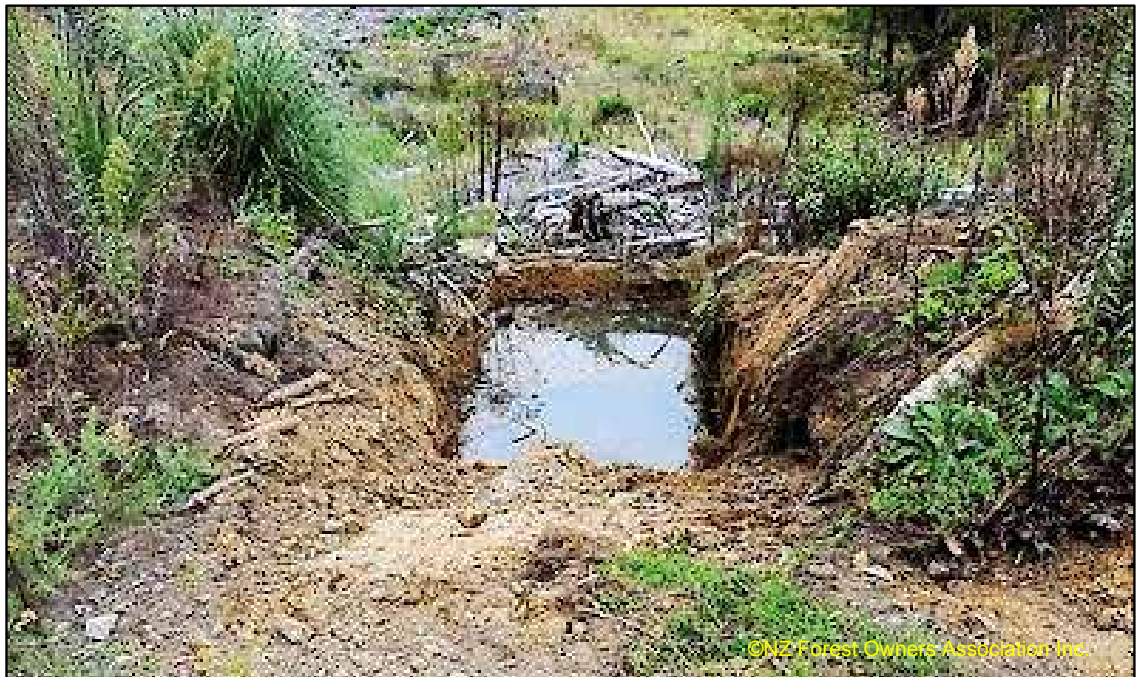
Figure 31: Sediment trap at skid trail - road junction
