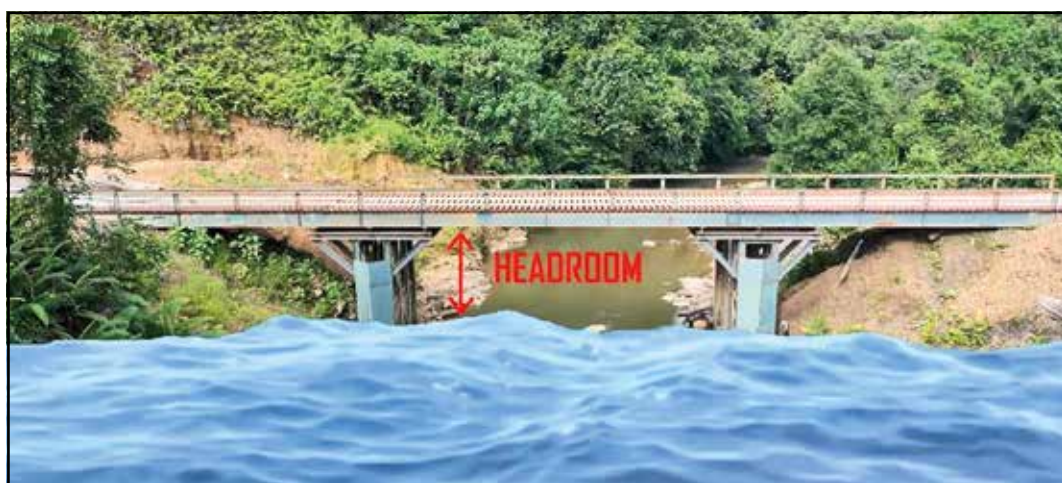
Figure 13: Adequate headroom between river flood level and the underside deck
