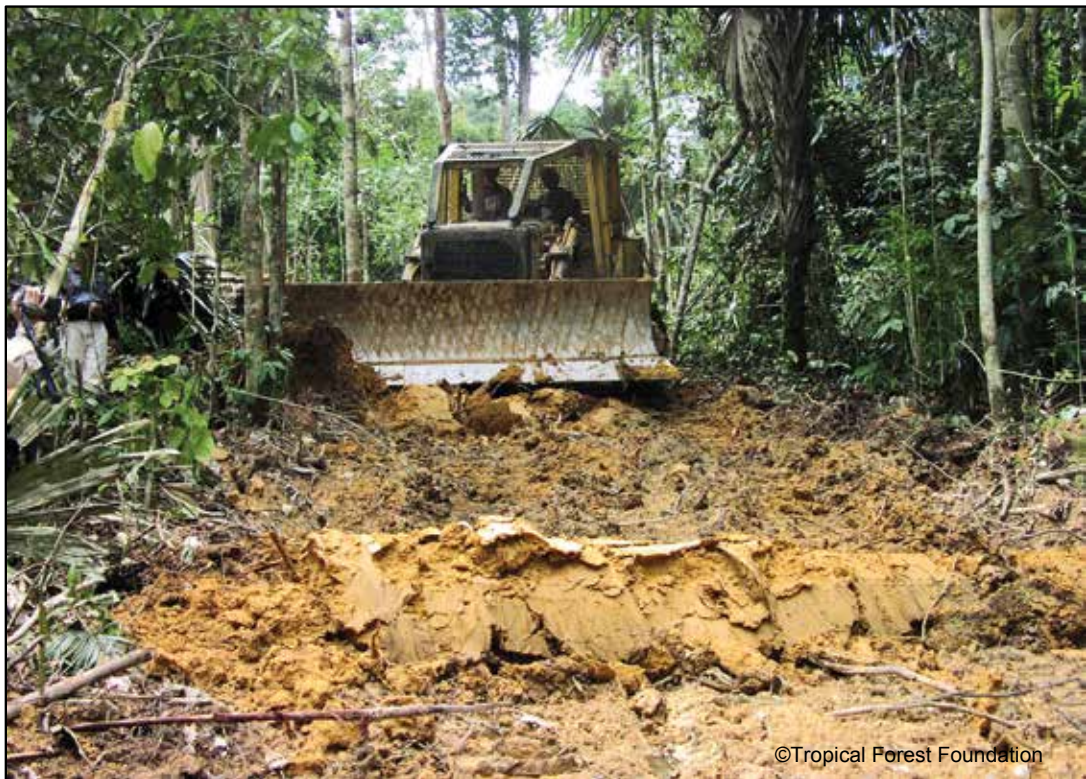
Figure 30: Cross-drain diverting skid trail runoff to vegetated area
