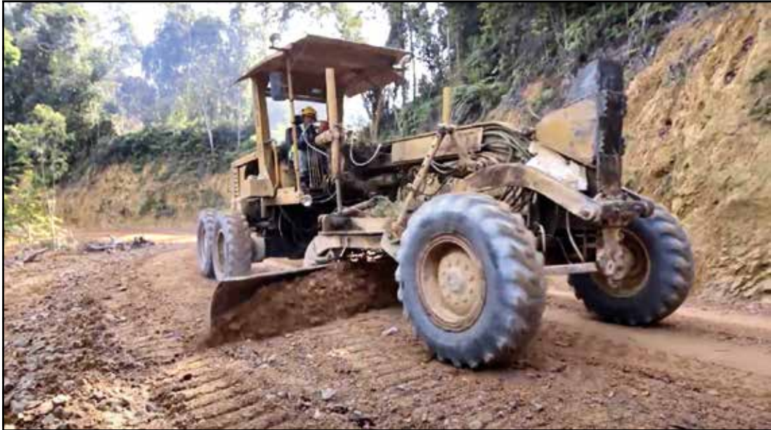
Figure 15: Road works with motor grader
