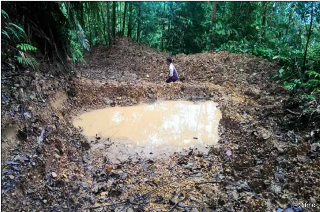
Figure 29: Water bump blocking skid trail runoff
