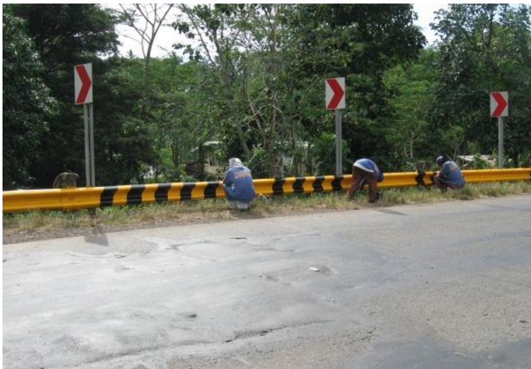
Road Maintenance - Painting of railings along the Iligan-Cagayan de Oro-Butuan Road
