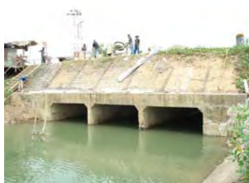
Culvert in the drain parallel to the Floodway
