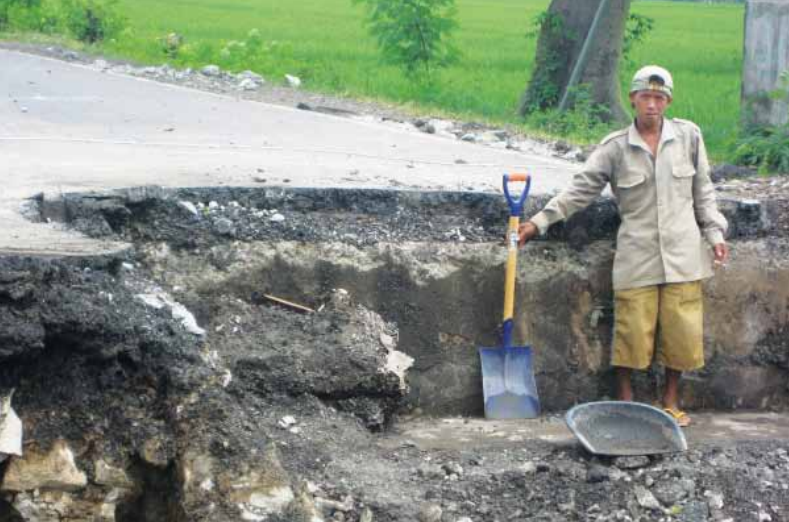
A cross-section along the Ciasem-Pamanukan section of the National Highway where a drain is being replaced. This project is part of a performance-based contract being operated on a pilot basis. Courtesy of Theuns Henning
