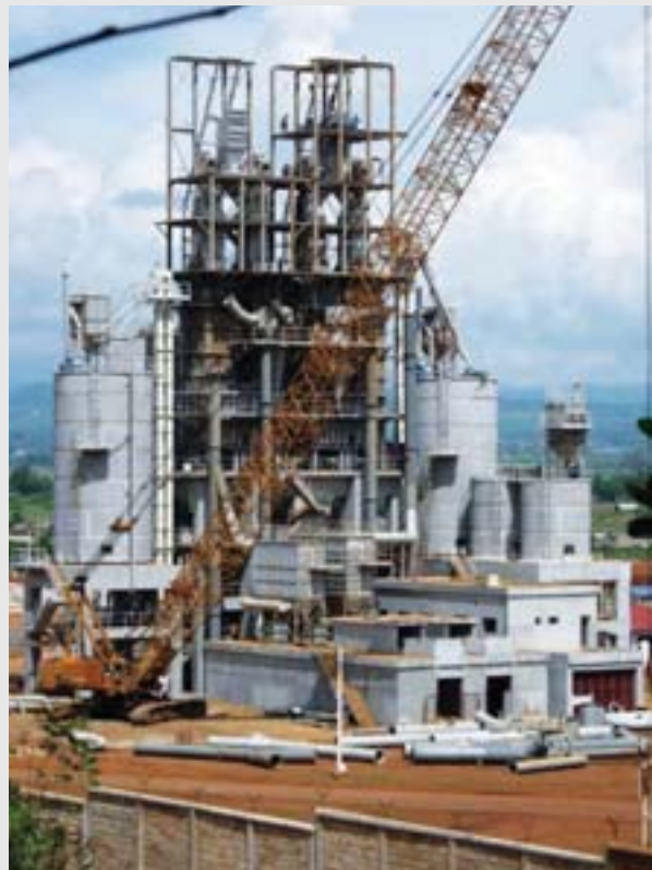
Pinpet iron factory under construction
