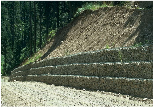
Figure 4.7 : Gabion in talus slope for consolidation
