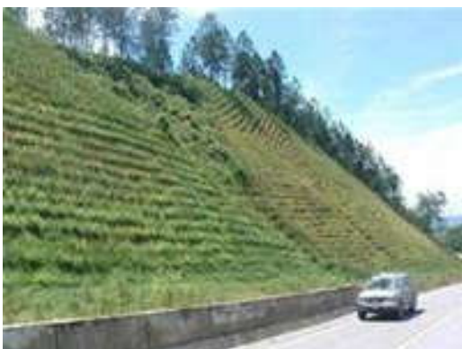
Figure 4.6 : Vetiver grass grows on Ho Chi Minh road, increasing stability of slop and create landscape
