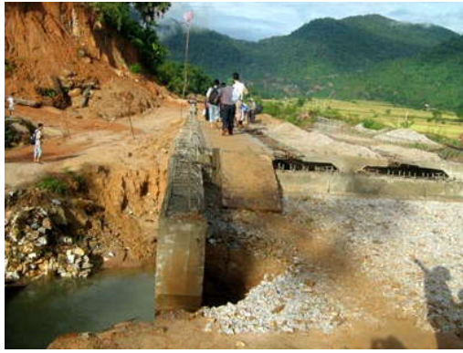
Photo 3.5 (Tông Đậu 08/2007). Flood take away embankment part and approach road of culvert when it is under construction.
