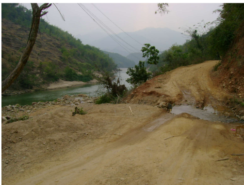
Photo 2.20: Water flow from top mountain crossing road surface, it's a factor to make erosion.
