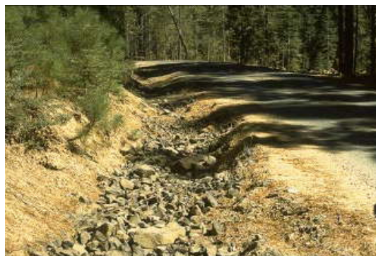
Figure 4.3 : Consolidate ditch by rock
