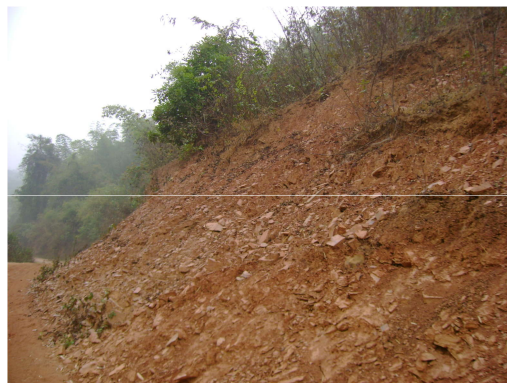
Photo 2.16: 30m Sliding of upper slope at ending section
