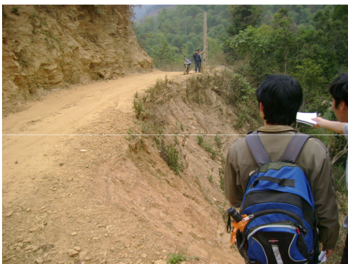
Photo 2.13: High degree slope with none consolidation, geography is claydy and laterite that unstable in rain reason
