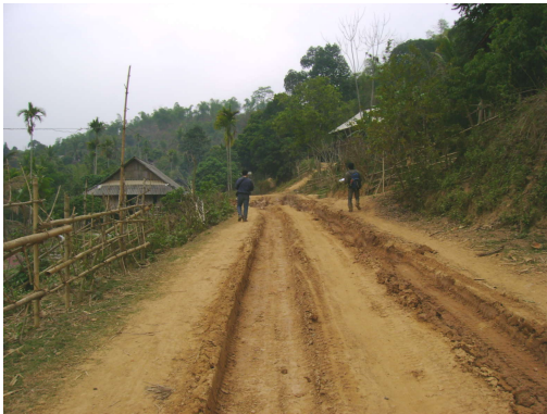
Photo 2.21: Serious damage of road surface, making difficult for traffic. Road services level low.
