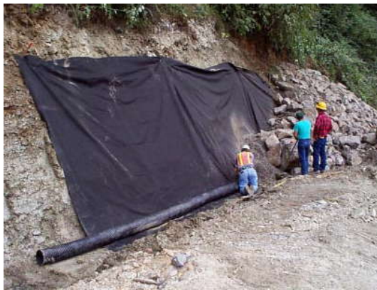
Figure 4.8 : Geotextile for increasing slope stability and avoiding erosion
