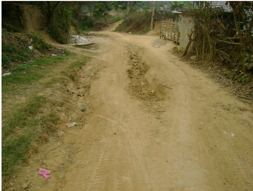
Photo 2.19: Excavation foundation but no side ditch. Water over flow to make erosion
