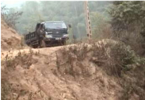
Photo 2.22: Bendy limited of vision, no protection, damage for vehicle
