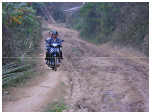
Photo 2.17: Road surface to be erosion due to over flow water
