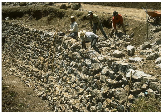
Figure 4.12: Using masonry revetment to reinforce talus slope
