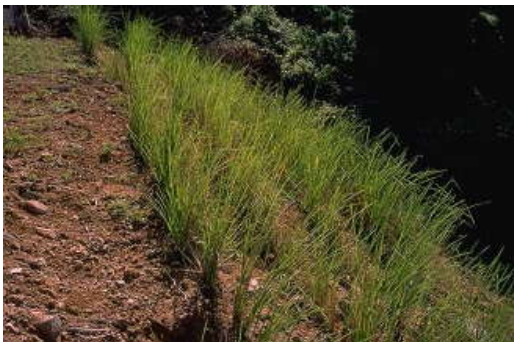
Figure 4.5 : Sodding on talus slop to enhance stability of slope and landscape
