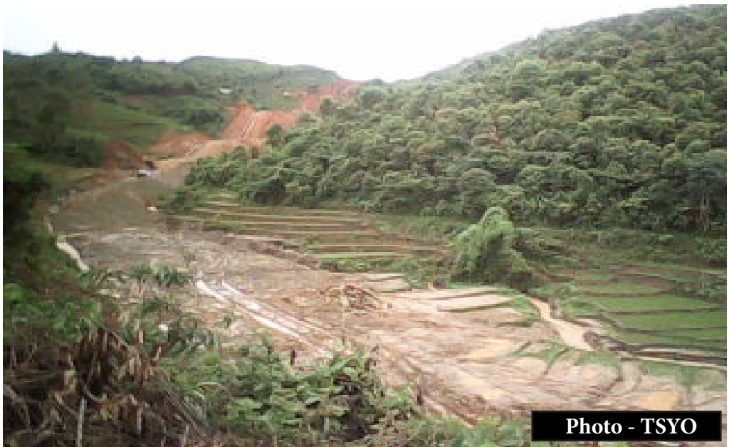
Raw sand from the drains of the pipeline flows to the paddy fieldsand destroys the paddy
