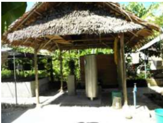
Figure 17. Pressure tank for water supply. ©KFI
