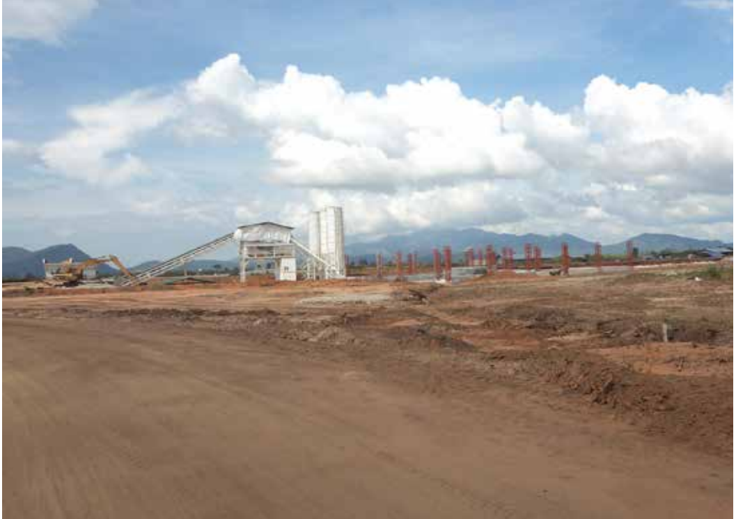
Project construction near Ngapidat village
