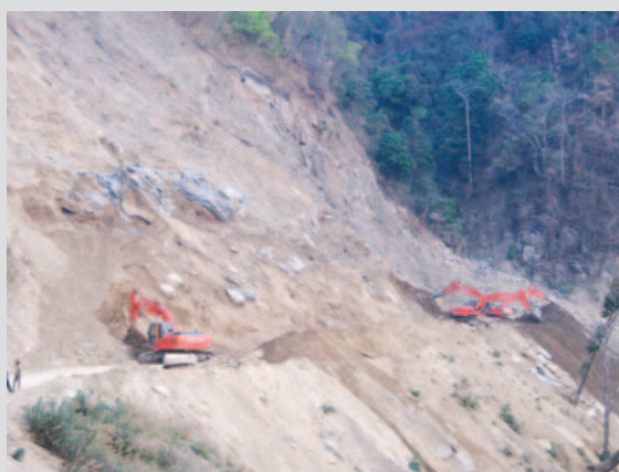
The highway construction passes through steep terrain
