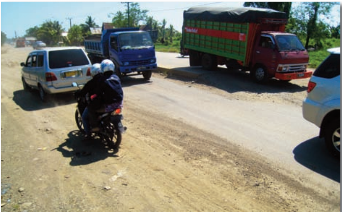
An absolute lack of signs at a work site in South Sulawesi. Notice that vehicles are driving on both sides of the road.
