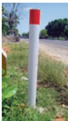
A plastic guide post – a low cost idea from the Fact Finding Mission to Melbourne in April 2010
