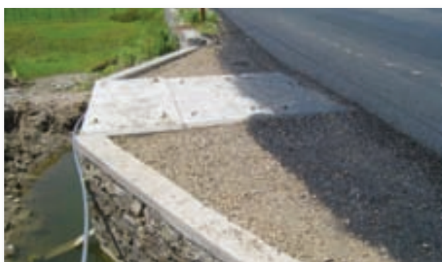
A culvert that has been extended in Central java. The further a hazard is relocated from the road, the lower the overall risk of the road.
