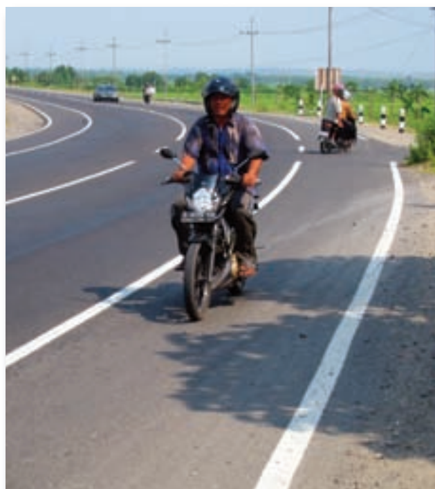
An example of a sealed shoulder – welcomed by motorcyclists and great to minimise the risk of vehicles running off the road. The sealed shoulder helps to maintain the road, and it eliminates dangerous drop offs.
