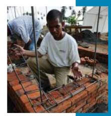
MERCY Malaysia's core houses were built with seismic-resistant technology
