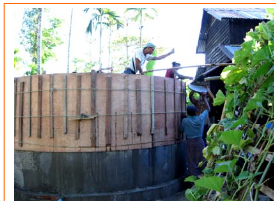
A concrete tank being constructed in Mawlamyinegyun township. The tank has a storage capacity to provide safe drinking water to 1,300 households. (Photo: MRCS)
