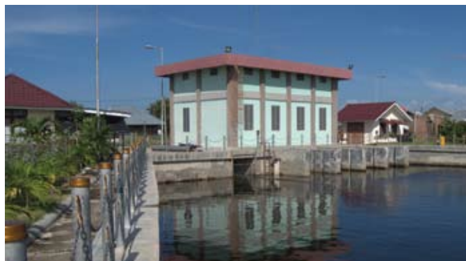
The Lampaseh water pump station helps keep the streets dry in Banda Aceh. The BAFMP project constructed flood gates and pumping stations to protect the flood-prone city.
