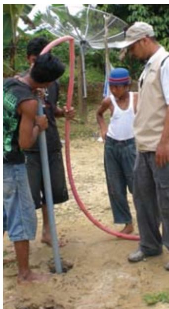
Community members install a water pipe for an artesian well in Simeulue. Grants from the CSO project were used to improve community facilities and to strengthen the capacity of local CSOs and CBOs in Aceh and Nias. PHOTO: UNDP COLLECTION
