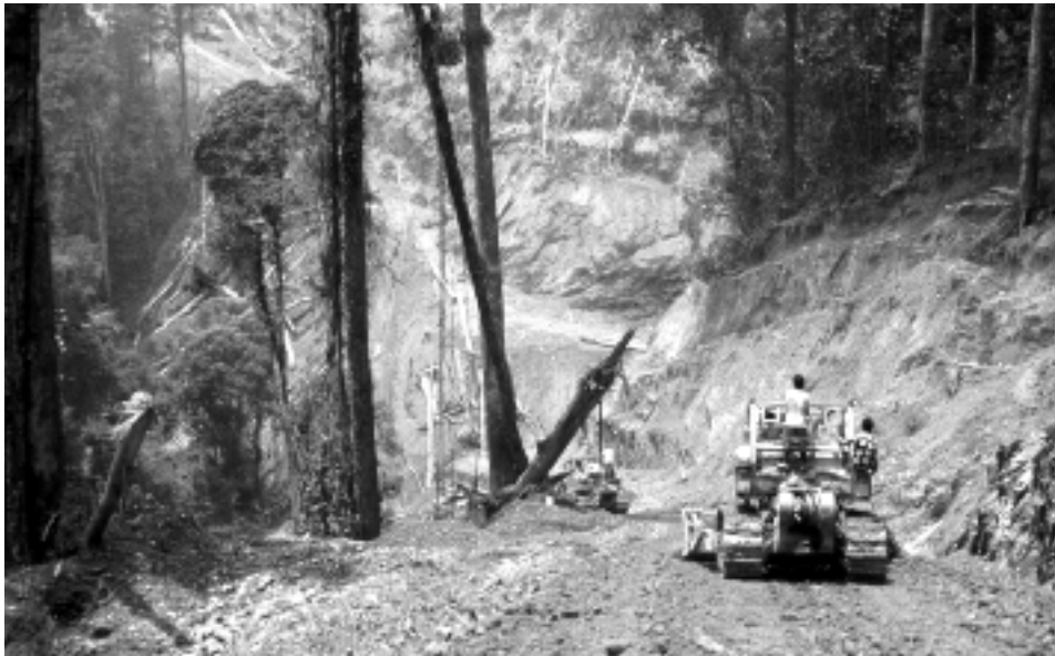
Figure 22. Logging roads are often unnecessarily wide, increasing the effects of forest fragmentation by inhibiting animal dispersal and increasing sedimentation levels and erosion. (Photo by Rob Fimbel)
