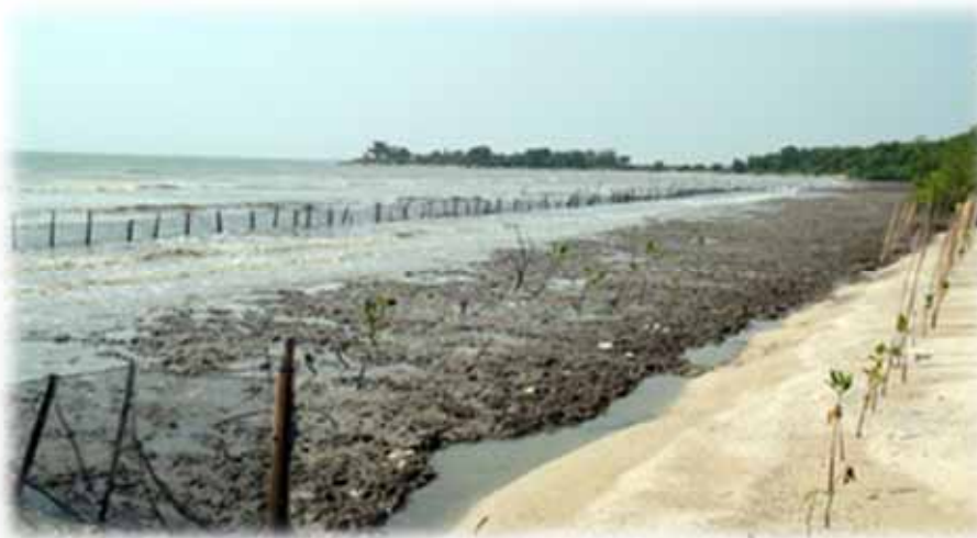
Figures 213. Condition of Area where Mud Trap Has been Constructed, after High Tide
