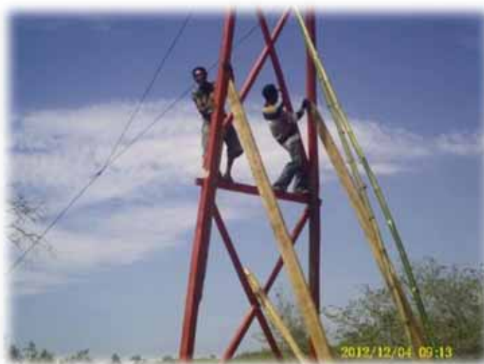
Figure 217. Construction of Observation Tower in Desa Darat Pantai.
