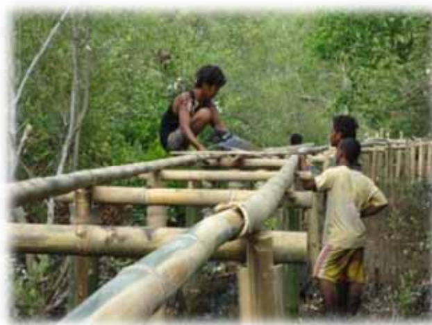
Figure 215. Constructing the Mangrove Track in Desa Reroroja.
