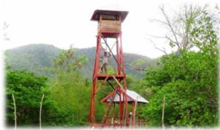
Figures 218. Observation Tower in Desa Darat Pantai.
