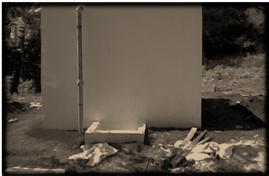
A PDC reservoir being constructed
