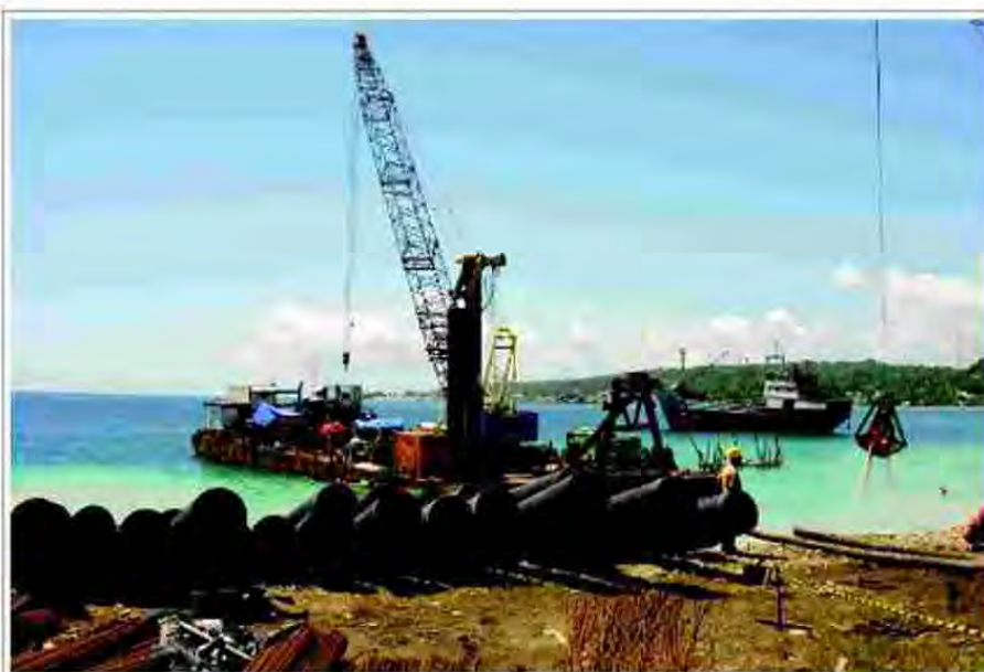
The Gunung Sitoli Port design under implementation. (Foto/Nis. S)
