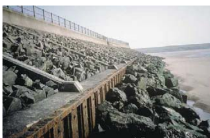
An example of revetment (Source: http://www.snh.org.uk/publications/on-line/heritagemanagement/erosion/appendix_1.16.shtml )
