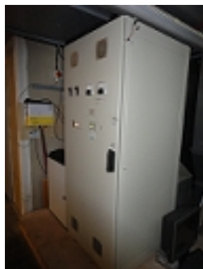
Fig.8. 5 Project Edison, the AC-DC converter and battery management controller.
