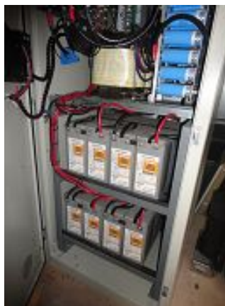
Fig.8. 7 Project Edison, the battery storage.
