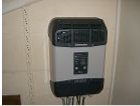
Fig.8. 17 The combined inverter and charger unit.
