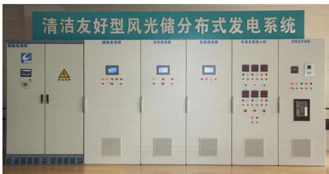
Fig.5. 10 Clean-friendly Wind-photovoltaic-energy-storage Distributed Power Generation System
