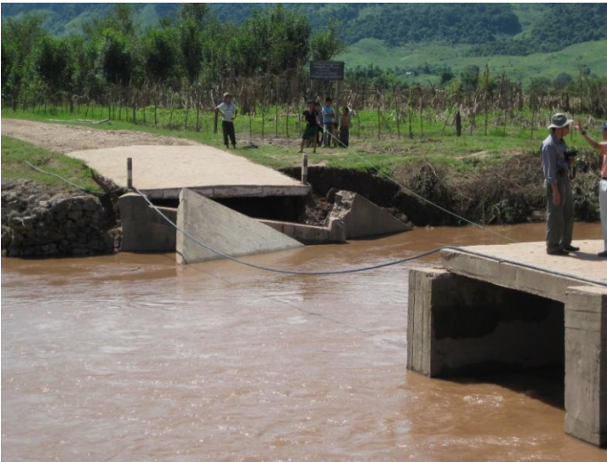
Figure 12: A completely damaged bridge in Xiengkhouang Province
