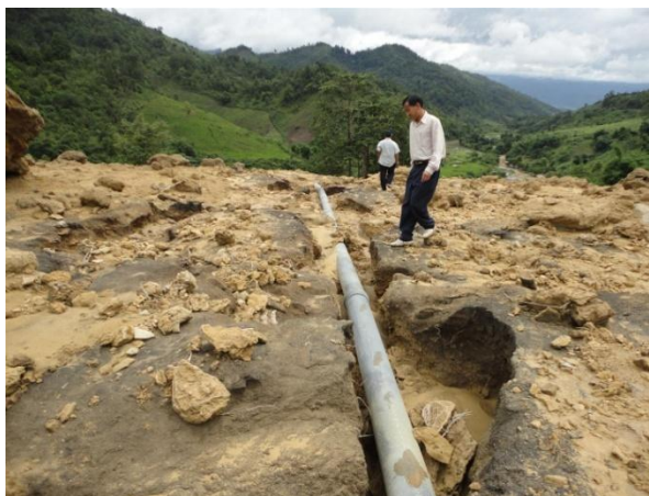
Image 9: Damage to Water Intake no.2 Khoun District, Xiengkhouang Province
