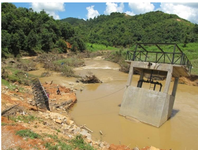
Image 9: Damage to Water Intake no.2 Khoun District, Xiengkhouang Province
