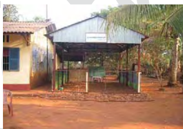
CLC at Village 14, Chub Rubber Plantation. The roof was of plastic material before; with funds from the Project, it has been changed to GI sheets
