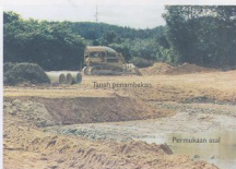
Rajah 2: Proses perataan tanah
