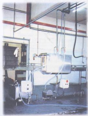
Plate 1 : Rinse water recycle system for floor washing and other cleaning purposes
