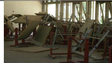
Becora Carpentry Workshop
