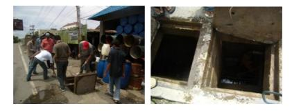
PS and Manhole (MH) construction was noted to be cast in place reinforced concrete, and the quality of construction appeared to be very good. No leakage was noted into the structures inspected. MH and PS hatches were noted to be steel framed reinforced concrete, and their removal required significant effort by 2 men.
