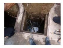
CAPACITY BUILDING FOR BANJARMASIN, BALIKPAPAN, AND SURAKARTA WASTEWATER EXPANSION UNDER INDII WATER AND SANITATION HIBAH Pump control for all PS is manual and at the local control center only. Level detectors in the PS appear to be on strings/cables in vertical pipes (floats or sensors), and are said to be for clean water use. All are non-functional at all PS in all areas.
