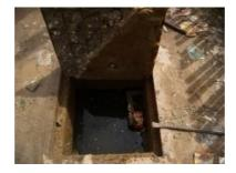
At another manhole, which was one of the manholes constructed of precast concrete components, the concrete manhole cover broke when a prybar was used to try to lift it. There was no rebar in the broken piece, indicating that the manhole covers are not properly made. Again the manhole was full of water. It is doubtful that the manhole has been constructed properly. Need to recommend design standards be implemented in all future DPU work throughout Indonesia.
