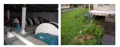
Figure 2.14. Basiri RBC STP System and Service Area
