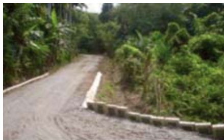
Road Reconstruction Phase III: Installation of Side Panels
