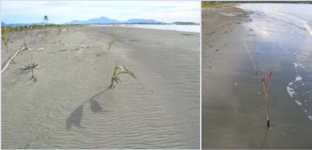
Figure 80. Abrasion in desa Kahju village
