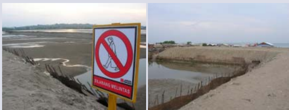
Figure 72. Almost completed embankment sea defence on mudflats at Desa Kedau Aceh village -Lhokseumawe
