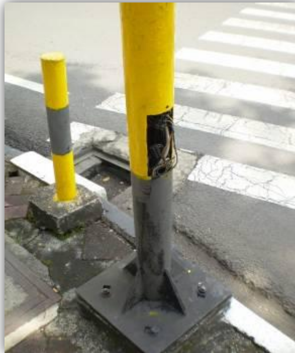
Figure 10: A pedestal with terminal strip cover missing, with exposed wiring
