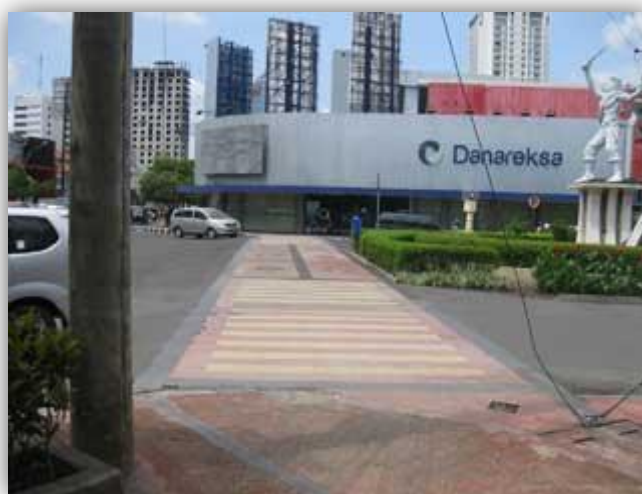
Figure 40: An example of a recently implemented raised pedestrian secondary road crossing
