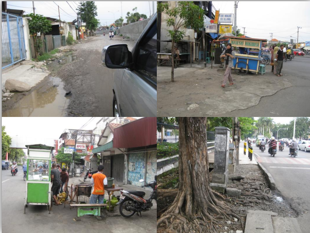
Figure 43: Broken drains, encroachment by vehicles and a crossing that leads nowhere
