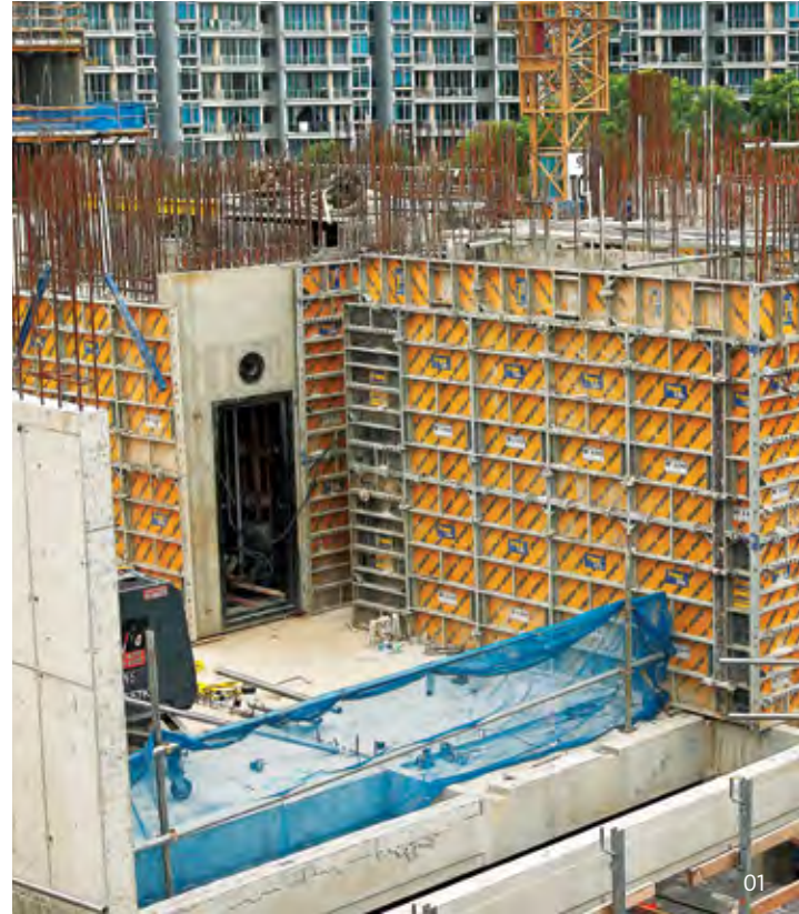
01 Use of system formwork in lieu of traditional formwork to improve site efficiency | 02 Raising the skills and capability of the workforce is crucial in realising the vision of higher productivity | 03 Drywall installation eliminates wet trades and speeds up construction
