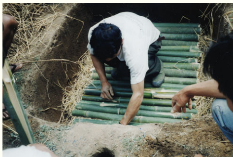
Laying bamboo segments at the kiln base
