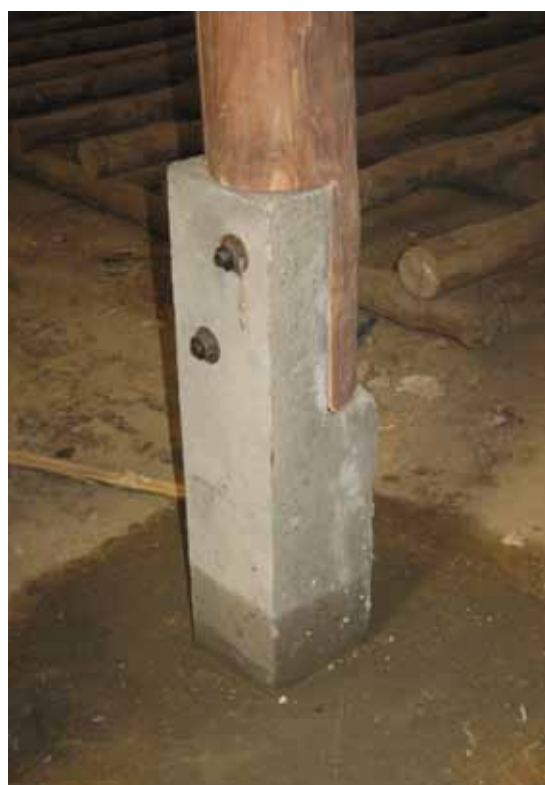
Concrete post foundations
