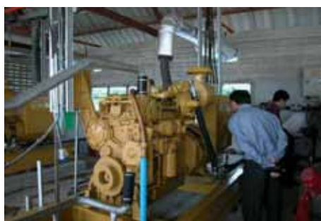
Biogas operated gas engines produce electricity from the gas produced in the covered lagoon Source: www.thaibiogas.net
