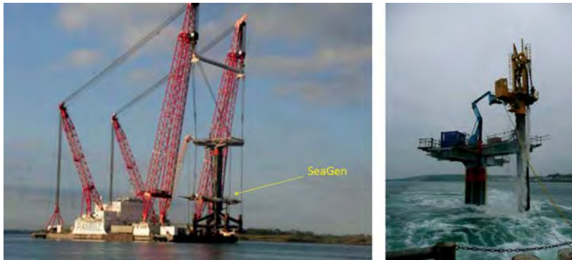
Figure 13. Crane Barge Rambiz arriving in Strangford Lough in late March 2008 to commence the installation of SeaGen (left). Drilling and grouting operations, carried out from temporary work platform (right)
