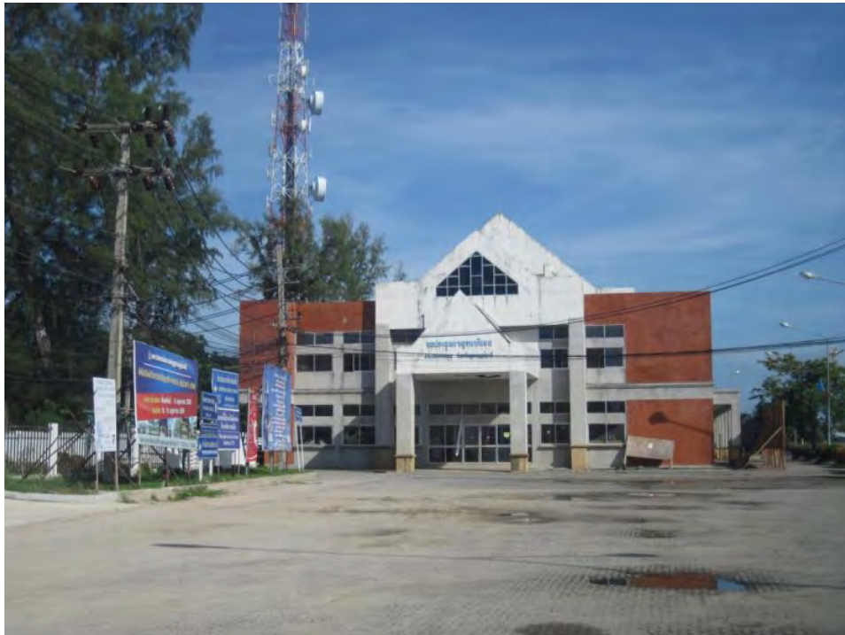
FIGURE 5-10: Kanchanapisek Conference Hall before proposed renovation
