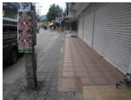
FIGURE 5-91: Uneven, poorly maintained and inconsistent walkways on Chaweng 1 Road
