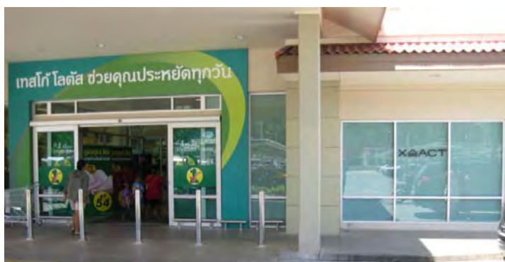
FIGURE 12-12 : Entrance of Tesco Lotus in SAMUI Island
