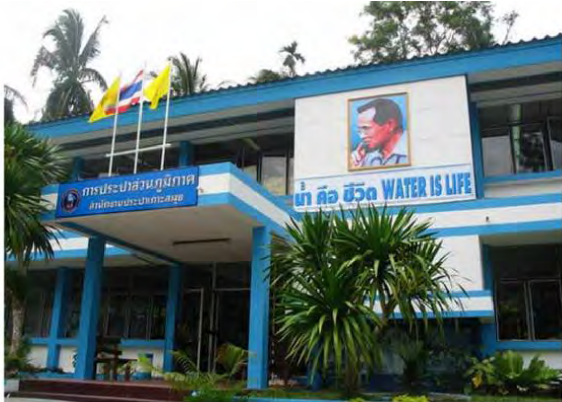
FIGURE 9-28 : Provincial Waterworks Authority of SAMUI Island.
