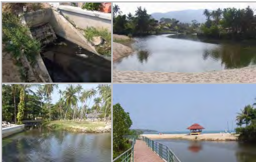
FIGURE 13-11 : Existing wastewater discharge point
