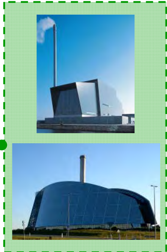
The New incinerator power plant
