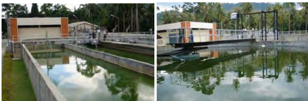
FIGURE 13-23 : Lamai - Hau Thanon Wastewater treatment plant
