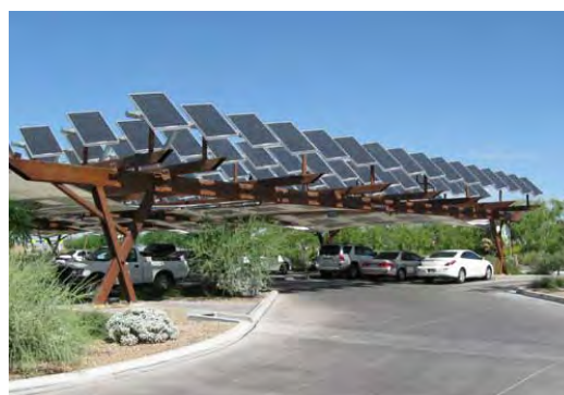
FIGURE 6-18 : Example of characteristic designed roof with PV
