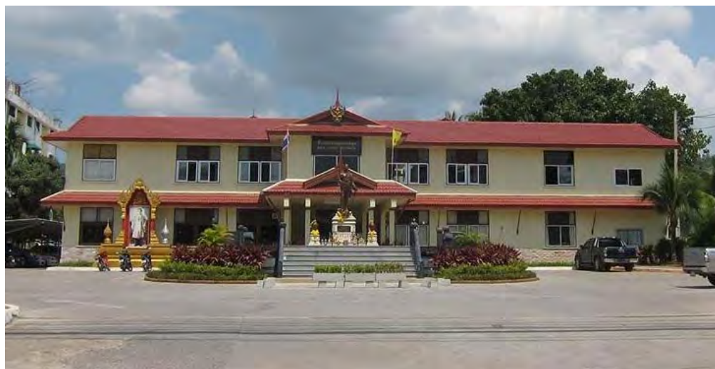
FIGURE 11-18 : SAMUI District Office
