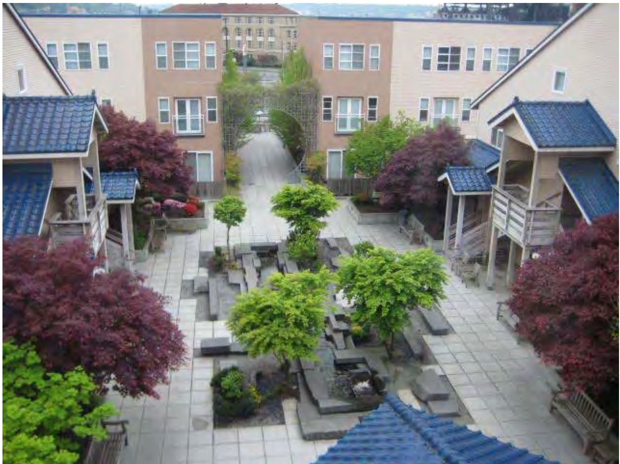
FIGURE 5-69: Uwajimaya Village Apartment, Seattle, USA
