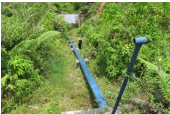
The penstock and powerhouse of the 11 kW hydro plant at Palanggaran. Source: Ashden Website
