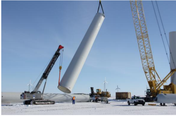
Figure 4. Installation of an EWT 900 wind turbine
