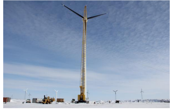
Figure 4. Installation of an EWT 900 wind turbine
